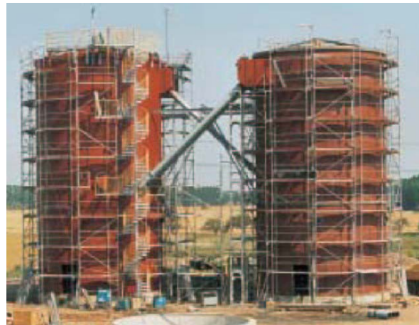
High capacity fermentation plants with a gas storage tank
